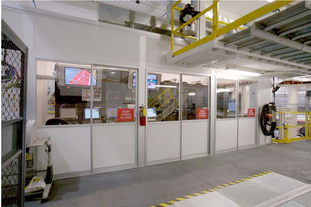
Figure 11. Phoenix Control Room.
